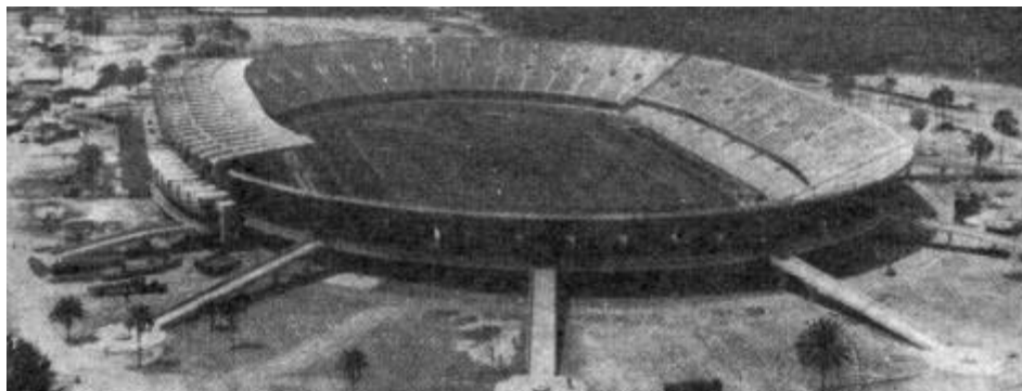
The national stadium at Lagos.
