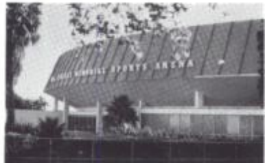
The Los Angeles Memorial Sports Arena, Los Angeles
