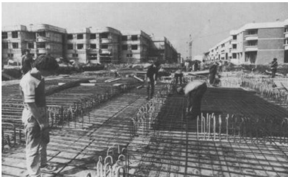
The Olympic Village under construction.
