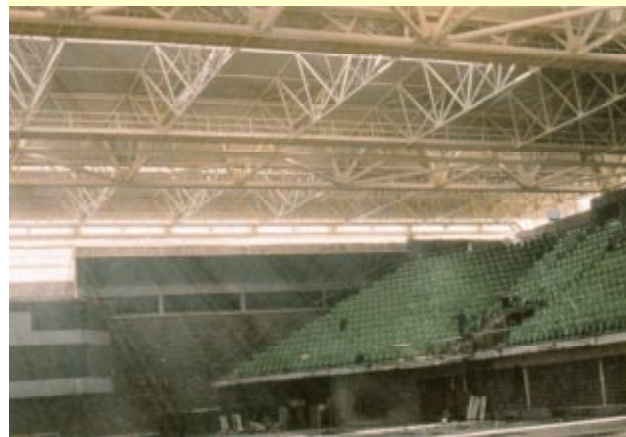
Inside view of the rebuilt Zetra Hall.
