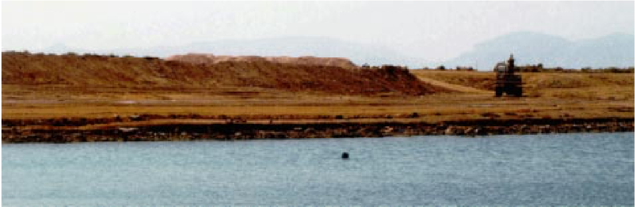
Beginning of the works in Aghios Kosmas, nautical centre and marina.
