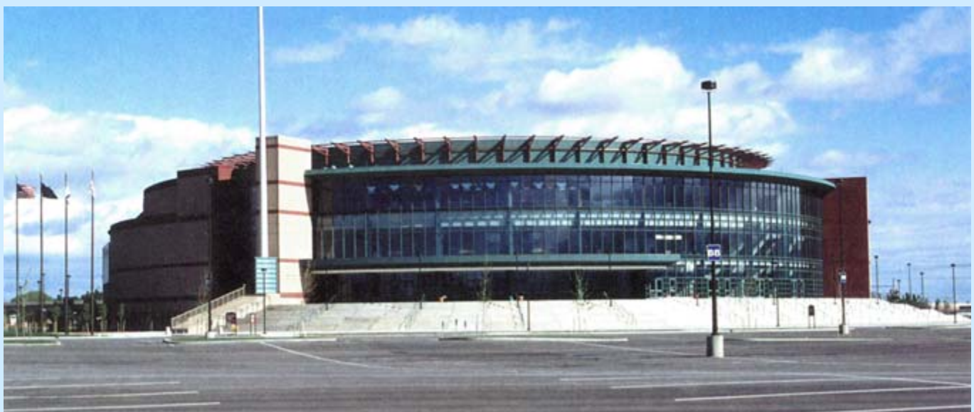
The E Center in West Valley City.
