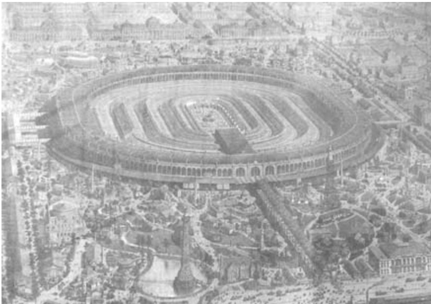
fig. 6: General view of the Paris exhibition of 1867, the exhibition building designed by Frédéric LE PLAY, in: Le Livre des Expositions Universelle 1857-1989 , Paris (Union Centrale des Arts Décoratifs) 1983, p. 220.
