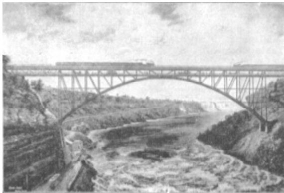
GRAND TRUNK RAILWAY'S SINGLE STEEL ARCHBRIDGE OVER NIAGARA RIVER.
