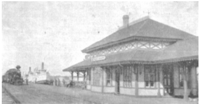
MUSKOKA WHARF STATION.
